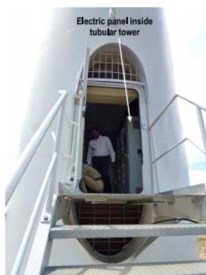
Figure 3.11 Tubular Tower Bottom: In a tubular tower, no separate building is required for the electric panel and transformer.
