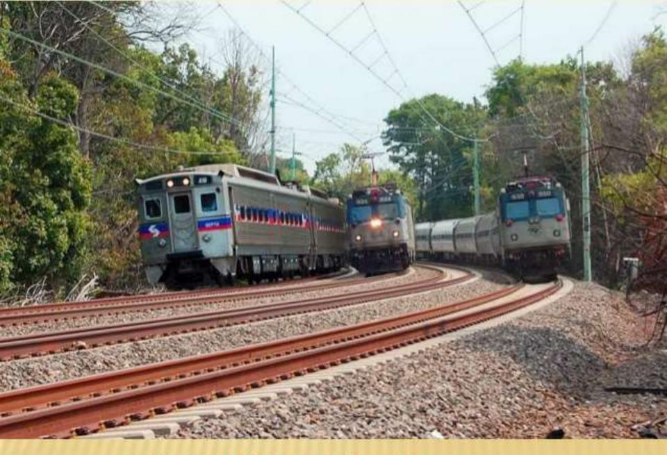
**Curve with superelevation**
