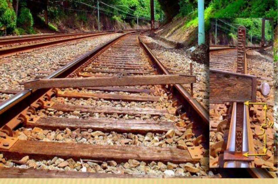
Superelevation between the inside and outside rails
